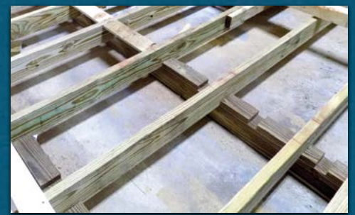
12" On-Center Floor Joists 16" OC is Standard
