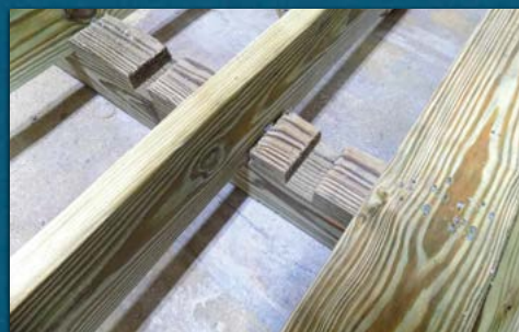
2x6 Pressure Treated Joists 2x4 are Standard
